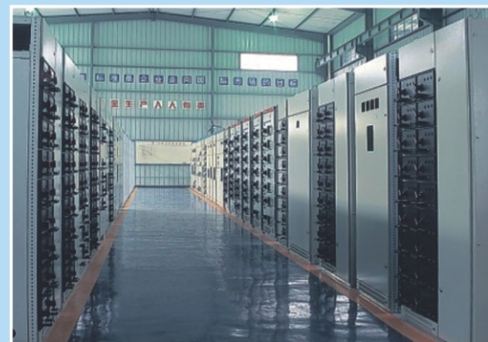
框架装配车间一角 Framework of the assembly shop
